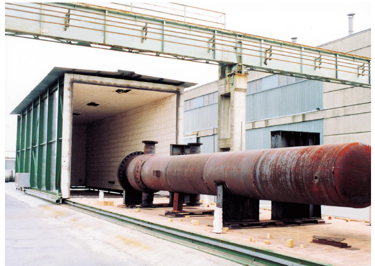
Gas fired Annealing Furnace for stress relieving of large vessels
