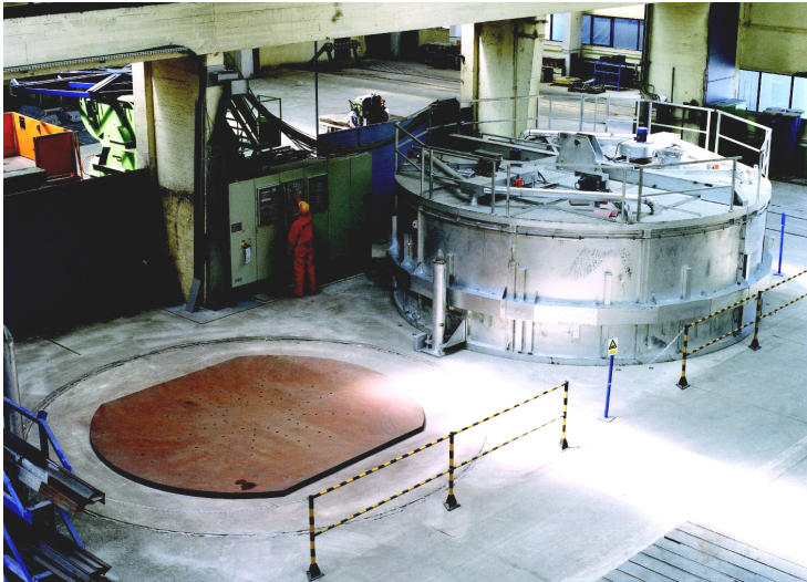
Electrically Heated Circular Kiln
